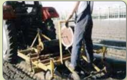
Laying down plastic (or similar) sheeting.
