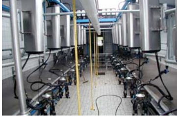
Milking parlour with a floor of tile
